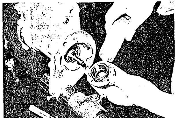
Applying BOND to bearing cover
